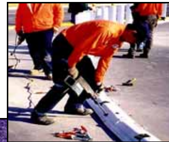
L60 Separator Unit 40" length 10 5/8 inch width 3 1/2 inch height
